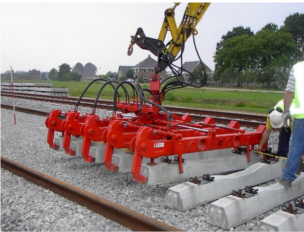
Apparatus for handling railroad ties
